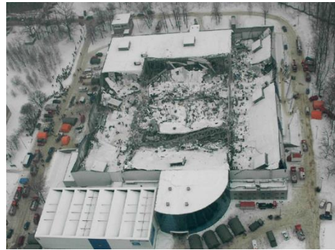
Figure 1. Roof collapse of Katowice Exhibition Hall
