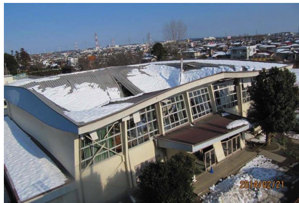
Photo 3. Example of collapsed building. (No.9 in Table 1.)
