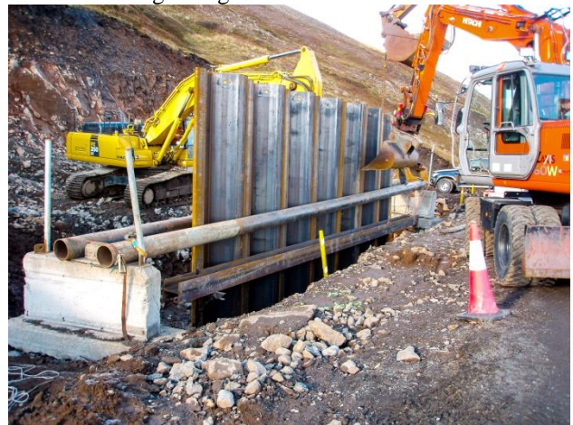
Figure 1. Installation of the steel sheet piles in 2011. Photo: IRCA
