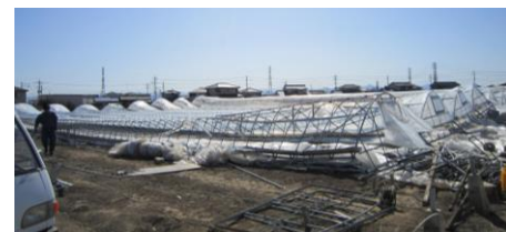
Figure 13. Collapse of a reinforced pipe-framed greenhouse due to snow load.
