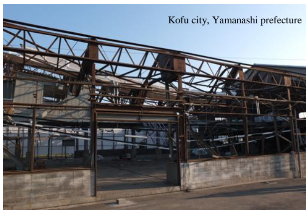
Fig. 1 Collapse of packhouse and equipment for packing
