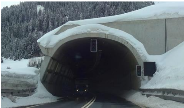
Figure 4. Entrance of the Cassanawald tunnel with portal collar in winter 2014, San Bernardino national highway. The width of the portal collar is 50 cm and the depth of the accumulated snow is about 80 cm.
