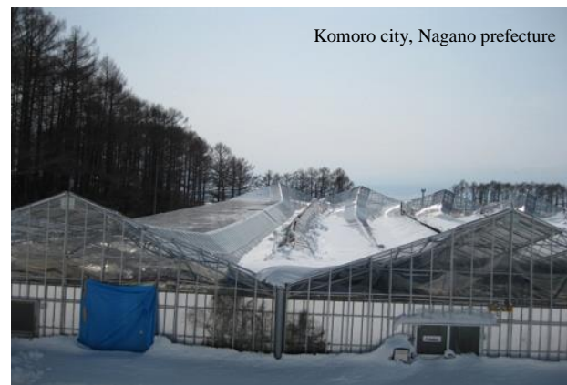
Fig. 2 Collapse of greenhouse due to excess snow load
