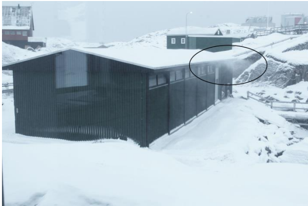
Figure 2 The tracing effect of snowdrift on a roof structure, Jennifer Fiebig 2015.
