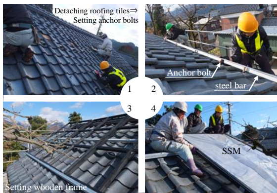
a) SSM installing procedure
