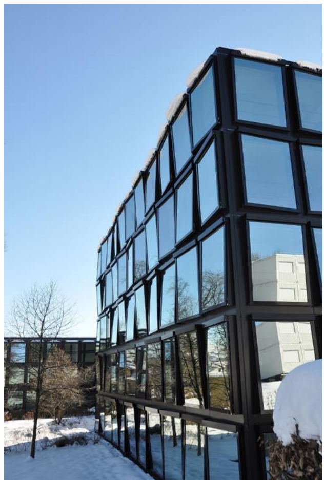
Figure 9. Snow accumulations on the window boxes of the existing Helvetia building on 10 February 2015.
