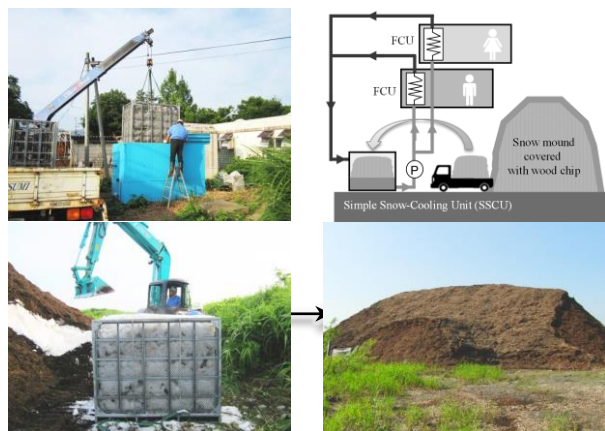
Figure 6. Snow cooling system for Highway SA lavatory.
