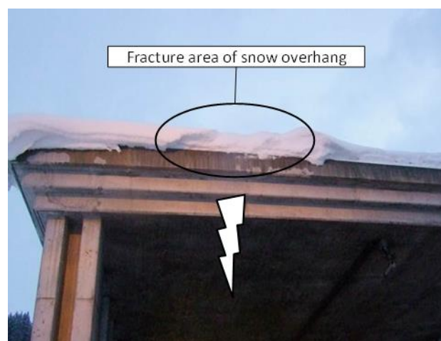
Figure 2. North entrance of the San Bernardino tunnel on 1 February 2014 with the fractured snow overhang (Photo Tiefbauamt Graubünden).
