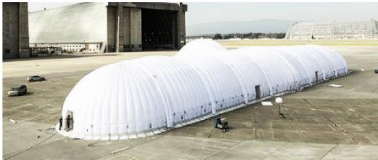
Figure 4: solar Impulse mobile hangar
